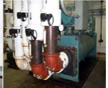
Chiller with Rusted Piping
